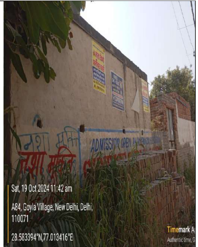
Pic 10. Boundary wall and house constructed on open channel
