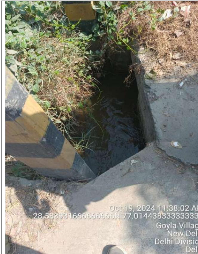
Pic 9. Waste-water discharge from drain leading into Najafgarh drain
